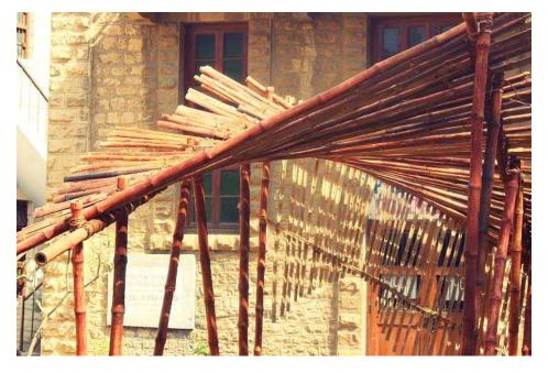
The two main materials used in this structure were Bamboo and Jute rope. Each bamboo was connected to the other with a traditional bamboo joinery technique 'lashing' using jute. Ar. Habibullah taught the students different lashing techniques which enabled them to avoid nailing in the structure. The bond
